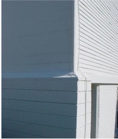
Wood flush board siding and clapboards
