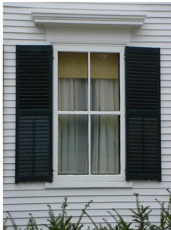
Well proportioned 2/2 light storm window over a 2/2 double-hung sash. In addition, the shutters are appropriately sized and placed.
